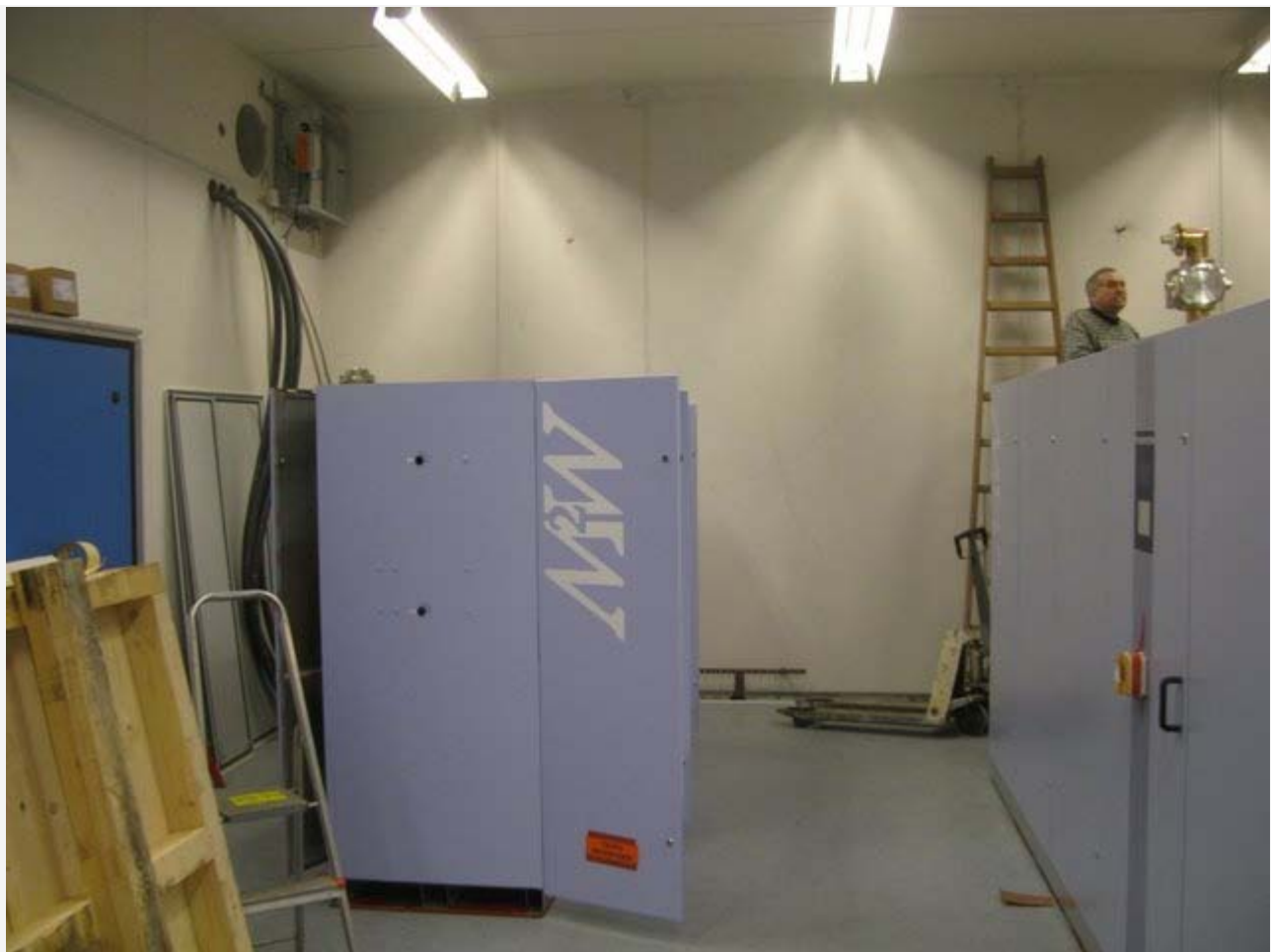
New 50kW and 100kW Thomson transmitters under installation
